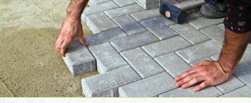
Clay brick pavers generally are considered more durable than concrete, and are ideal for warm weather climates that experience heavy sunlight. Because these bricks are solid in color all the way through, they won't show chips and scuffs as easily. However, clay brick pavers are typically more expensive and may not always be a financial option for some.
