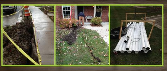
Drainage project in progress for condo residents where water was pooling in their yards. Our efforts required the need to boar beneath the sidewalks, and installation of sound pipe products.
